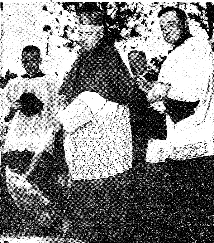
A spade full of dirt is turned by Bishop Coleman F. Carroll as work gets under way on the St. Thomas Catholic Student Center at the University of Miami, Coral Gables. The new building will serve as a spiritual and cultural center for Catholic faculty members and students of the university. The Bishop is flanked by Father Thomas L. McDermodt (left) and Father Thomas Anglin.
