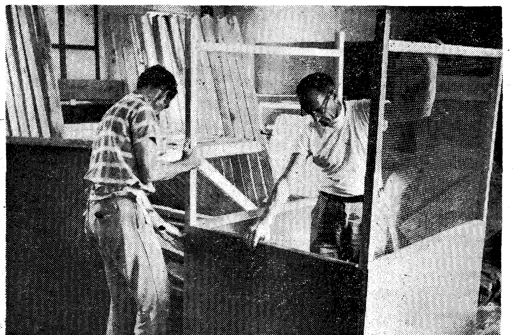
BUILDING BOOTHS where saleable items will be displayed requires the time and labor of men in the parish who donate many man-hours to construct and erect a large number of booths.
