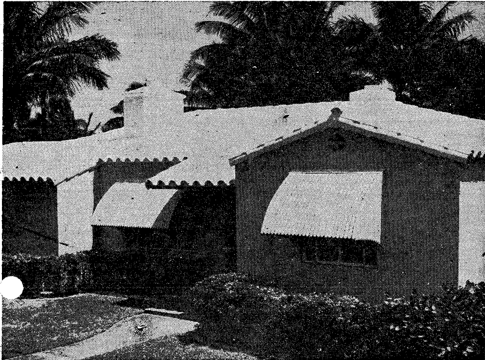
ALL JOINTS HAVE PURE BED OF WHITE CEMENT - FOR STORM PROTECTION
