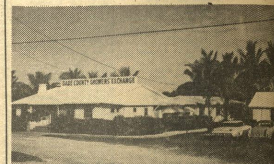
DADE COUNTY GROWER'S EXCHANGE-Roof recently cleaned & given TWO coats of lasting WHITE-TITE.
