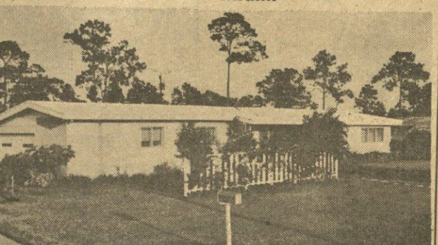
Mr and Mrs. M. H. McElmoyle, 11525 S.W. 69th Court. Sealing and coating of the gravel roof was completed more than 27 months ago.
