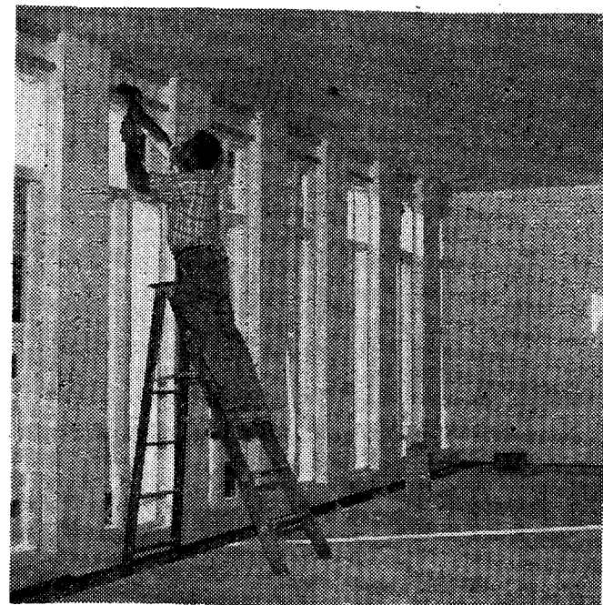
Windows in Hospital Chapel Will Be Set in Precast Frames
