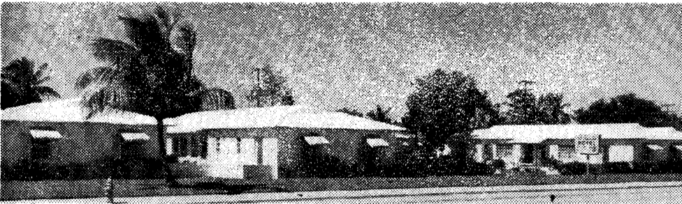
The El Shores Motel, owned by E. Mihalek, at 8840 N.E. 2nd Ave., Miami Shores, shows the matchless beauty of THERMOGLAZE coated roofs. THERMOGLAZE is an exclusive formula developed for GEORGE OBENOUR JR. & SONS, Inc.
