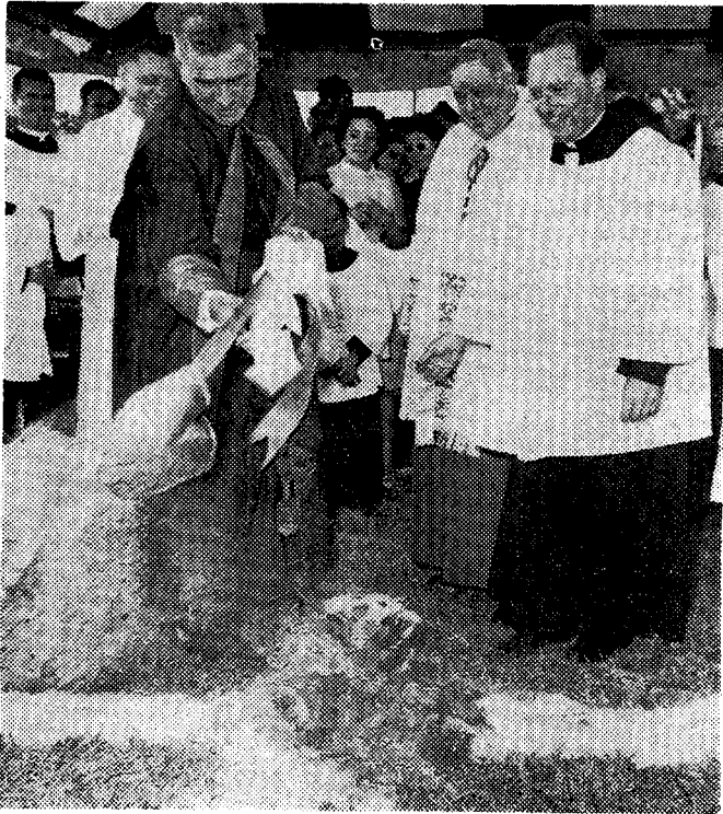
FIRST SHOVEL of earth to break ground for the new St. Michael Church was turned Sunday by Bishop Coleman F. Carroll assisted by Msgr. R. E. Philbin, former pastor, and Father Sebastian Loncar.
