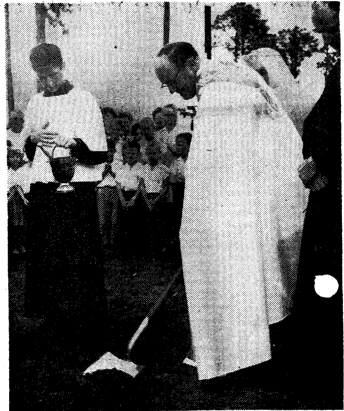
FIRST SHOVEL full of earth to break ground for a new wing at St. Charles Borromeo School, Port Charlotte, was recently turned by Father Xavier Morras, pastor. The addition will provide cafeteria, library, meeting room, and classroom.
