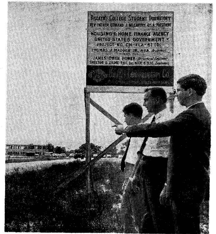
BISCAYNE COLLEGE'S new dormitory now under construction is pointed out by freshman, George Gerceo, Jr., of Philadelphia, to his father, and brother, Louis, after their arrival in Miami.
