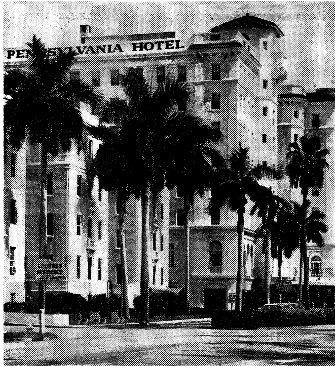
EIGHT-STORY retirement residence was formerly the Hotel Pennsylvania and adjoins the Lourdes Residence for the Aged. Both are staffed by the Carmelite Sisters for the Aged and Infirm whose motherhouse is located at Germantown, N.Y.
