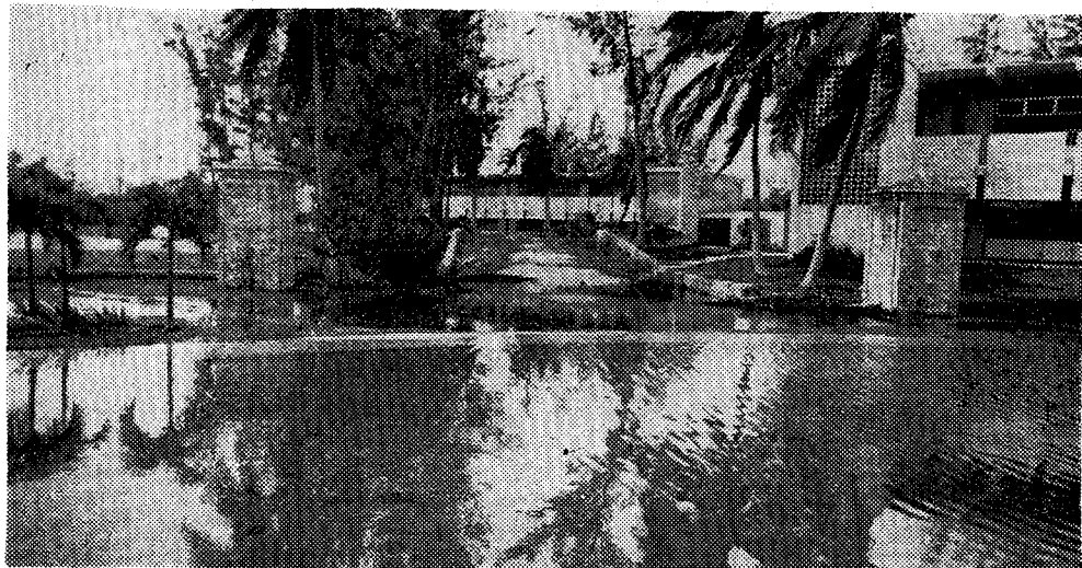
View Of Grounds At Immaculata-La Salle Academy Where Damage Was Heavy
