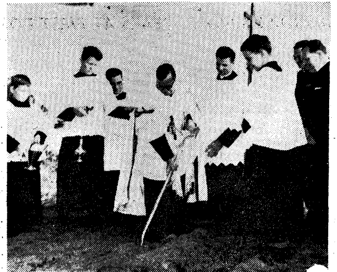
FIRST SHOVEL of earth to break ground for St. Cecelia Church was turned by Father John Neff during ceremonies on property adjoining Bishop Verot High School in Fort Myers. About 500 persons will be accommodated in the new church.
