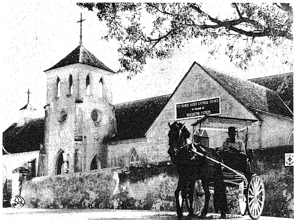
OLDEST CHURCH in the Bahamas is St. Francis Xavier
