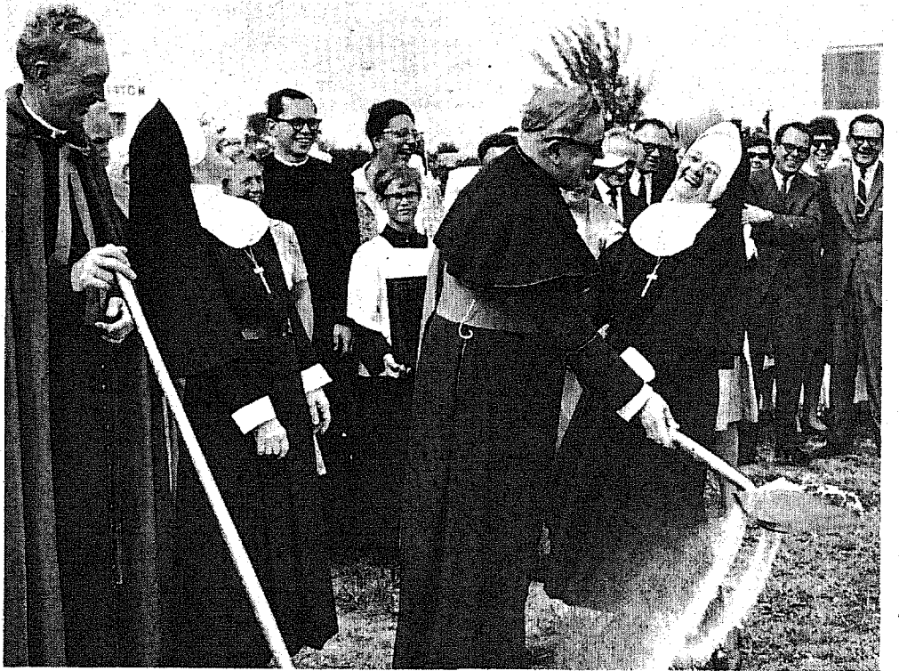
DIRT FLEW as ground was broken Saturday by BISHOP COLEMAN F. CARROLL and Sisters of Bon Secours for the new Villa Maria Nursing and Rehabilitation Center in North Miami. Shown with the Bishop are MOTHER FRANCIS HELEN, right, Villa Maria superior; MSGR. JAMES F. ENRIGHT, Vicar for Religious; and Mother Mary Alice, provincial superior of the Sisters of Bon Secours, at left.
