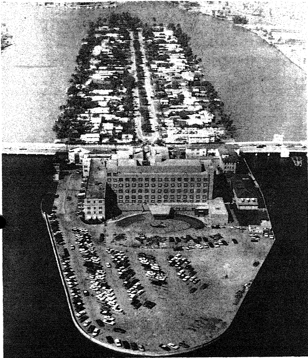
NEARING COMPLETION is the new wing at St. Francis Hospital, Miami Beach, which when opened will provide additional beds. Sisters of St. Francis of Allegany, N.Y. operate the hospital.
