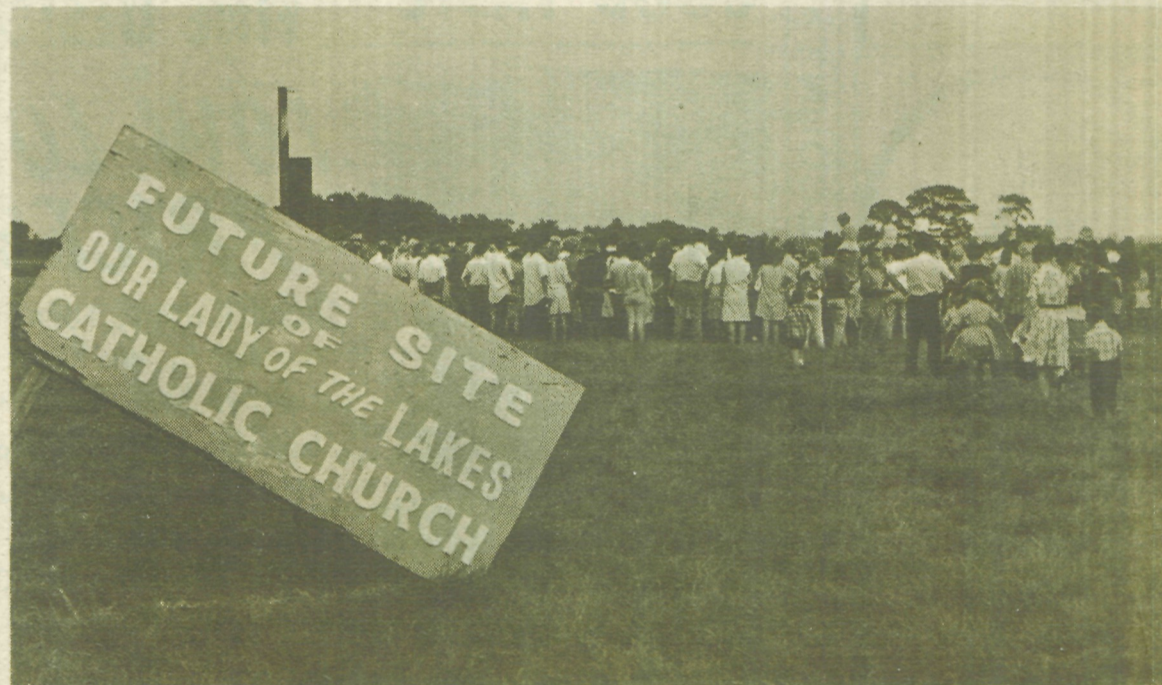
Ground Was Broken Sunday For Newest Church In Archdiocese.
