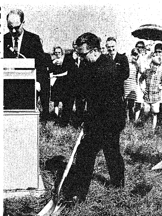
First shovel of earth to break ground for Our Lady of the Lakes parish center is turned by Father Miguel Goni, pastor.
