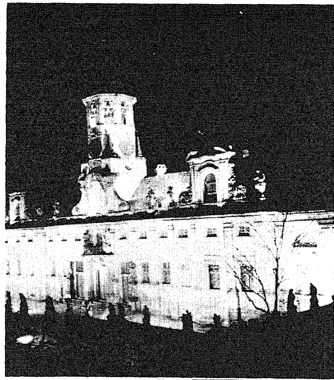
LORETO CHURCH , well lighted at night, has been one of the key tourist attractions in Prague. Built in 1661, the church was inspired by the Santa Casa in the Italian town of Loreto.
