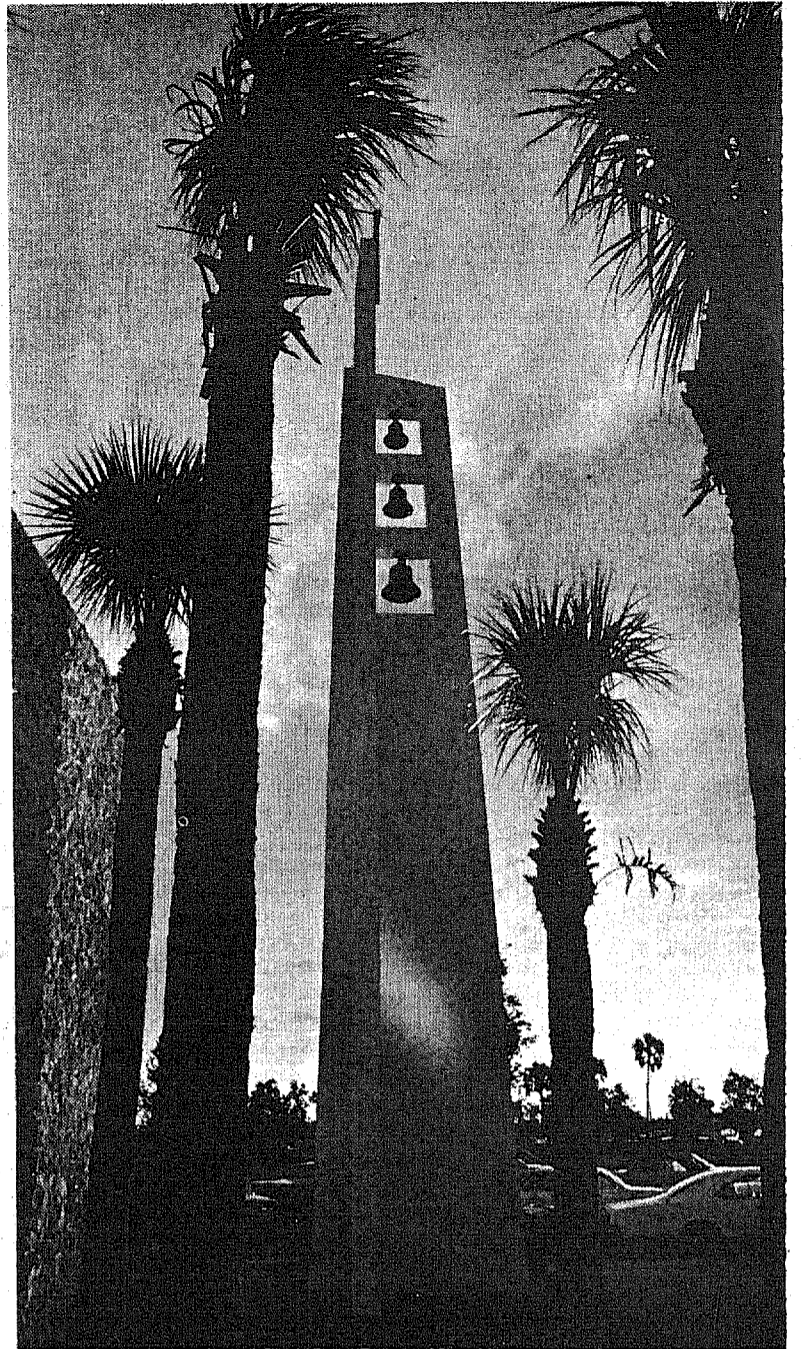
BELL TOWER of the new complex features three cast bronze bells which are electronically controlled.
