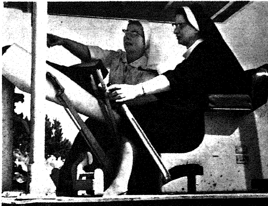
OPERATING BULLDOZER Mother Superior Louis Edwin, S.S.J., superior general of the Sisters of St. Joseph who operate Mercy Hospital, inaugurates construction of new buildings at the general hospital. Shown with her is Sister M. Emmanuel, S.S.J., executive vice president.
