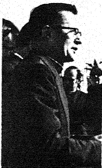
DURING ground-breaking ceremonies of St. John the Baptist Church, Father Thomas Dennehy, pastor, thanks parishioners and all those who have helped make the initial construction possible.
