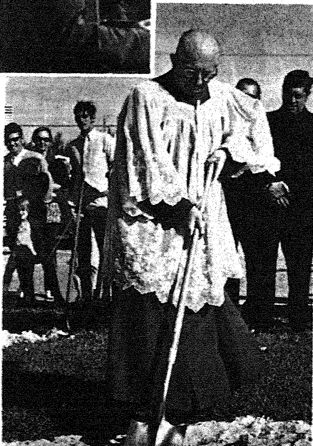
DIGGING UP the first shovel full of dirt, Msgr. John J. O'Looney, pastor of St. Anthony Parish in Fort Lauderdale, begins the first phase for the construction of the new St. John the Baptist Church. The church will be adjacent to Cardinal Gibbons High School. To the left of Msgr. O'Looney is Father Salvatore Profeta.
