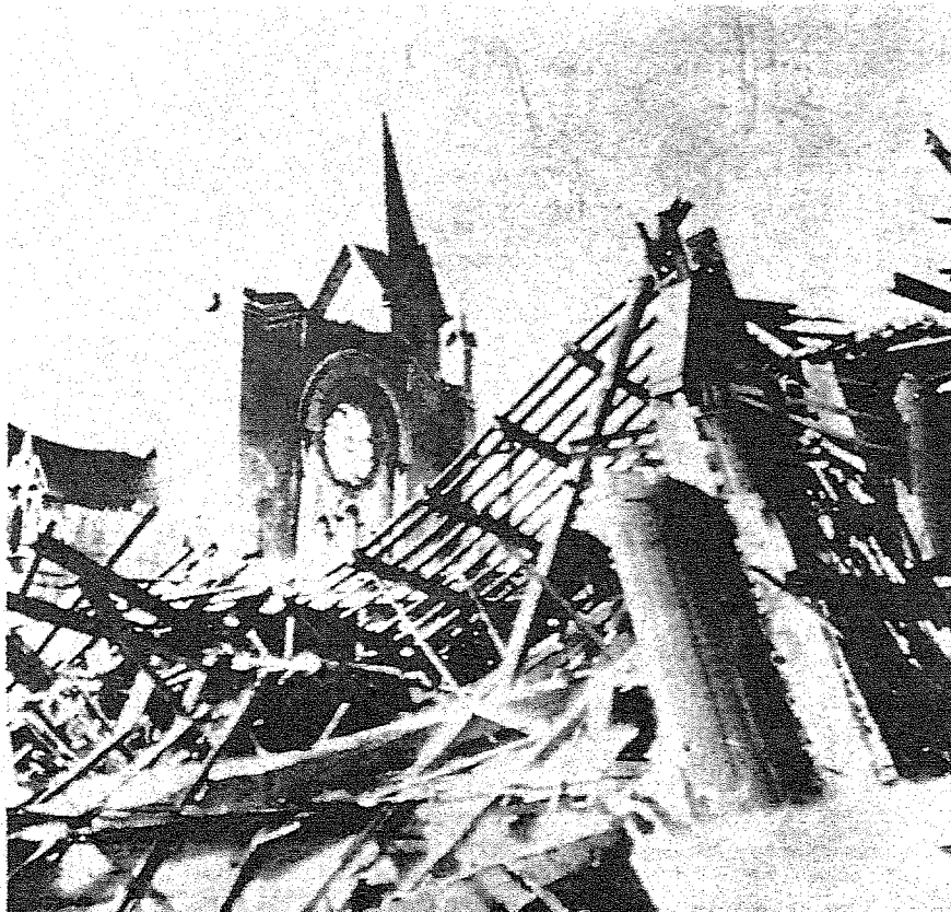
A CHURCH stands, amid the rubble in Managua. About 75 per cent of the city's buildings were destroyed in the disaster, and the rest have been declared unsafe. The government cut off food supplies to the survivors of the quakes to force them to leave before decaying bodies under the rubble caused an epidemic.
