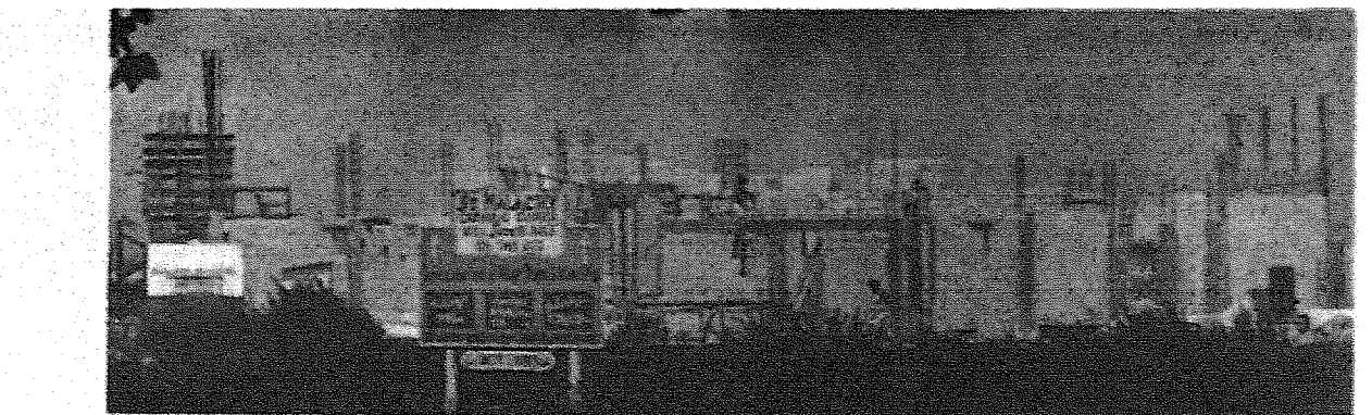
UNDER CONSTRUCTION in Fort Lauderdale is St. Malachy Parish Center designed by Miami architect Murray Blair Wright. Father Timothy G. Hannon is pastor of the Broward County parish, located at University Dr. and Bailey Rd.
