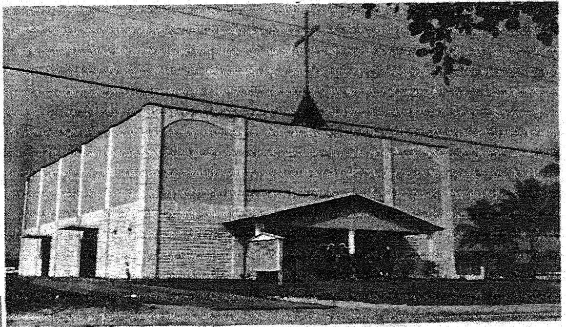
Ascension Multi-Purpose Center in Boca Raton.
