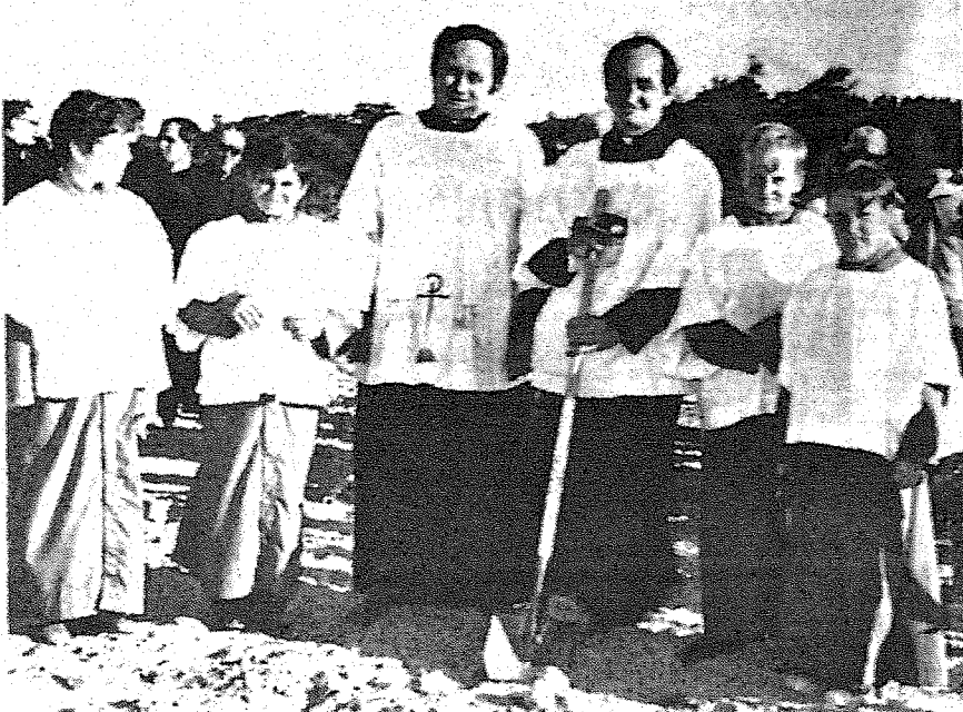
FIRST SHOVELS FULL of earth to break ground for St. Henry Church and multi-purpose center were turned in Pompano Beach by Father Brendan Grogan, pastor, right; and Father Patrick Murnane, V.F., pastor, St. Helen Church, Fort Lauderdale. The structure will be built at McNab Rd. and N. Andrews Ave.
