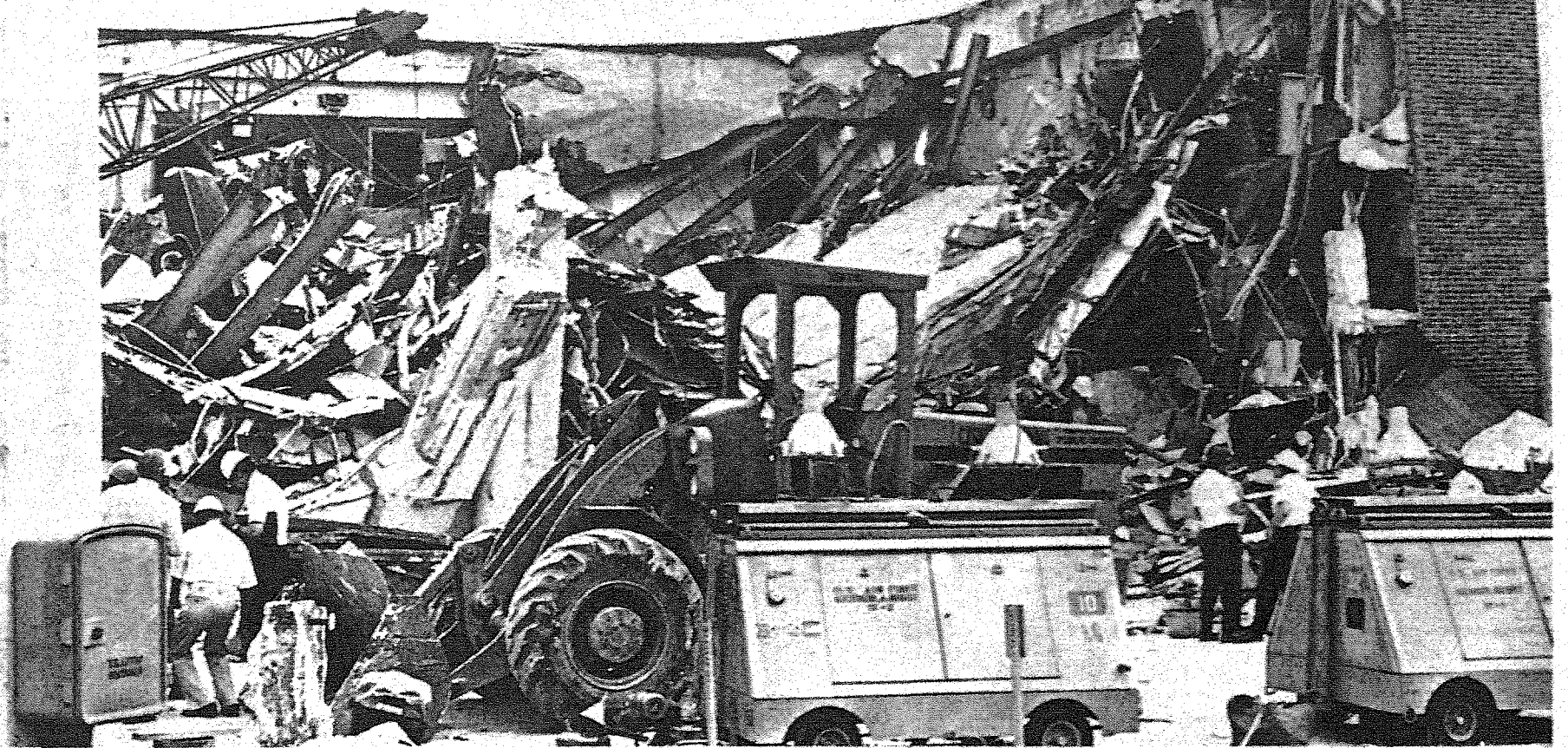
Twisted mass of concrete and metal injured 16 and killed 7 at drug agency headquarters .
