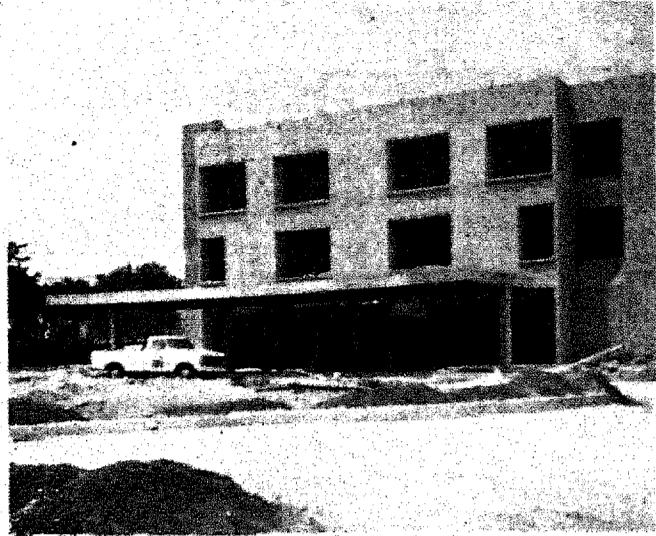
Exterior of Phase I of the construction on St. Mary's hospital shows work ahead of schedule, now set for completion in September.
