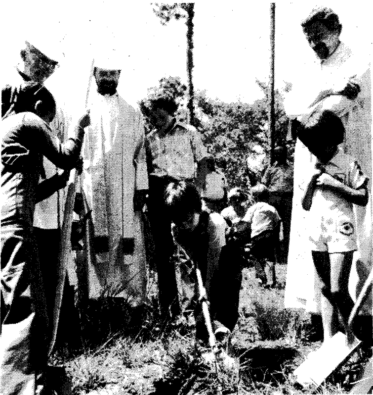
Children helped in groundbreaking ceremonies for a multi-purpose building at St. Richard parish last Sunday. Shown in background (L. to R.), are Msgr. John O'Dowd, V.F., Father Kieran Darcey, Administrator of St. Richards, and Father Roger Radloff.
