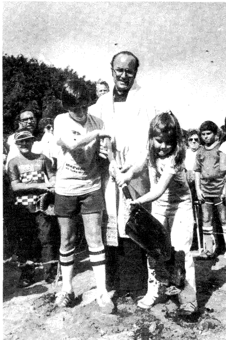
Helping hands are offered by two young parishioners, Chris Morro and Yvette Fierro, to Father Jose Luis Hernando, pastor, as the first spade of earth is removed for construction of the new St. Benedict Church.
