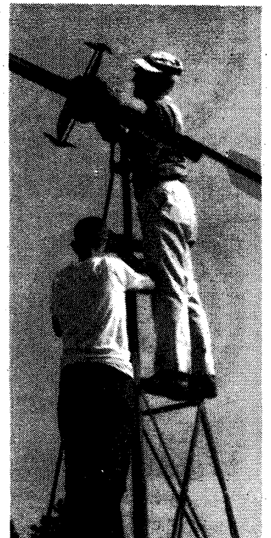
The E.D.C. has an Electrical Wind Generator (which powers our lights) and a windmill that pumps our well water to a reservoir located on the roof, which provides the water pressure for our entire system.
