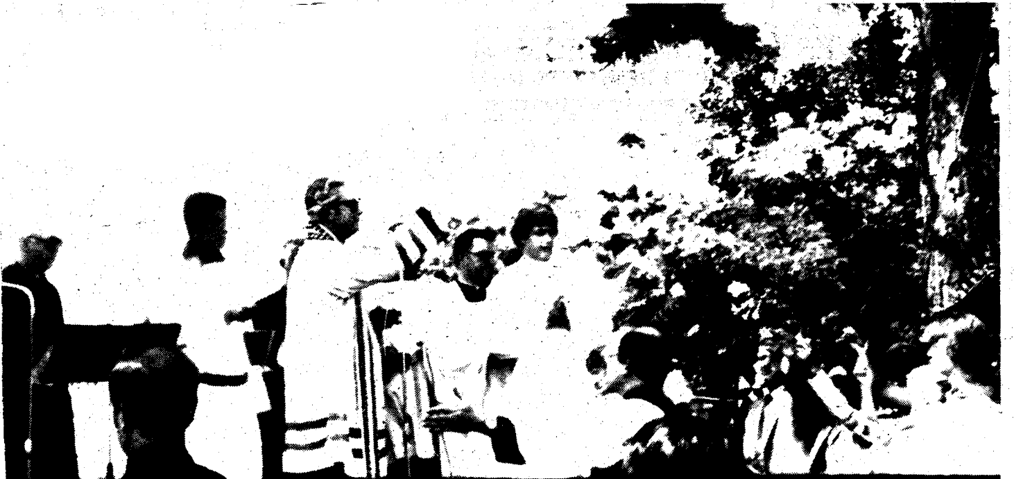
Site is blessed at groundbreaking as participants hold up holy oil vials.
