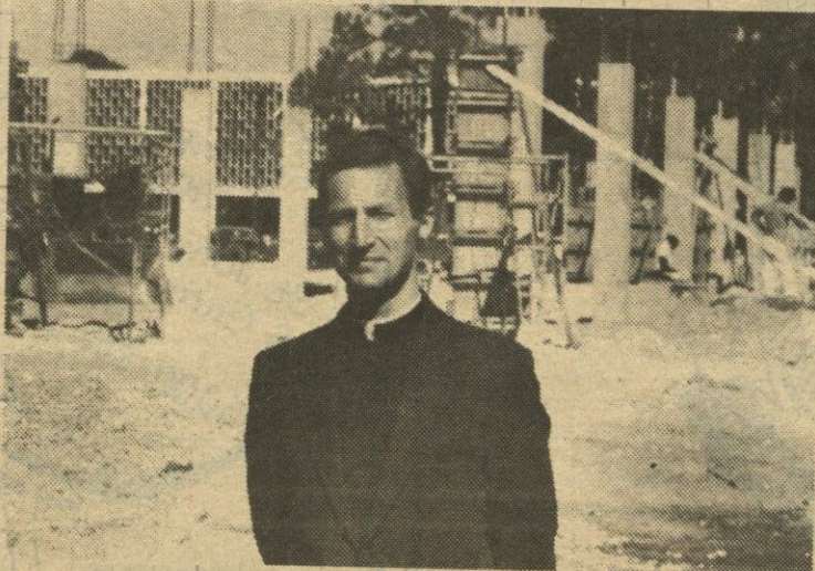
Fr. Pat O'Neill, President of Biscayne College, oversees construction of Biscayne's new $5 million Library, completion of which is slated for September, 1982.
