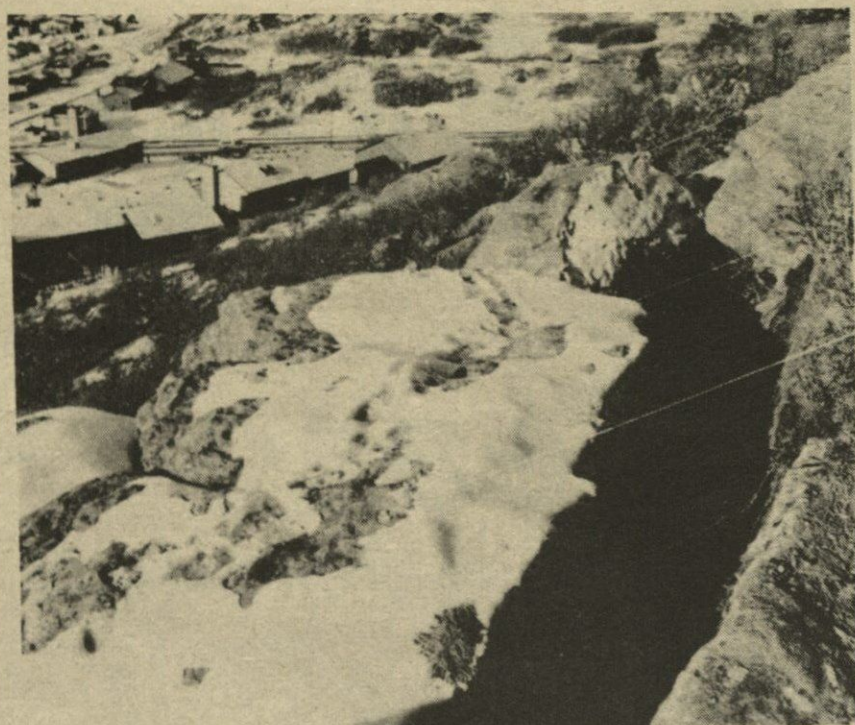
ROCK MENACE — A huge boulder hangs menacingly over subdivision homes in Castle Rock, Colo. Because the slipping boulder is on church property near St. Francis of Assisi Church, the Denver Archdiocese has been working with Castle Rock and Douglas County officials to dismantle and remove it. (NC Photo by James Vaca)
