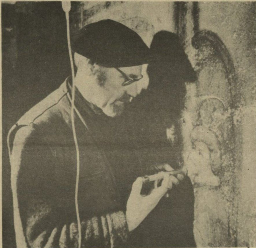
FIGHT AGAINST TIME — Restorer Friedrich Leonhardi fights against the tooth of time which gnaws at the 550 year old frieze of Bartholomaeus at the Frankfurt Cathedral. He uses a syringe and other medical instruments to fill hollow places that have formed under the plaster in the West German church.
