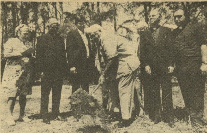
NEW RECTORY — The Church of the Resurrection of Our Lord, in Dania, recently had a groundbreaking ceremony for a parish administration center and rectory. Pictured are (left to right) Mrs. Ada Conti, Rev. Raoul Poirier, Robert Conner of Conro Construction, Tom Sette, Pres. of the Dania Chamber of Commerce (breaking ground), Richard Baker, architect, Fr. Joseph O'Connor O.S.A., pastor of Resurrection church and associate pastor Fr. Joseph Spinelli O.S.A.
