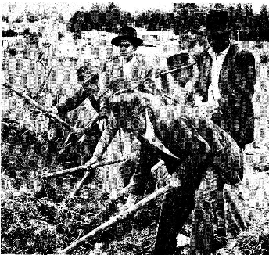
Peasants in Ecuador work diligently on a CRS construction project.
