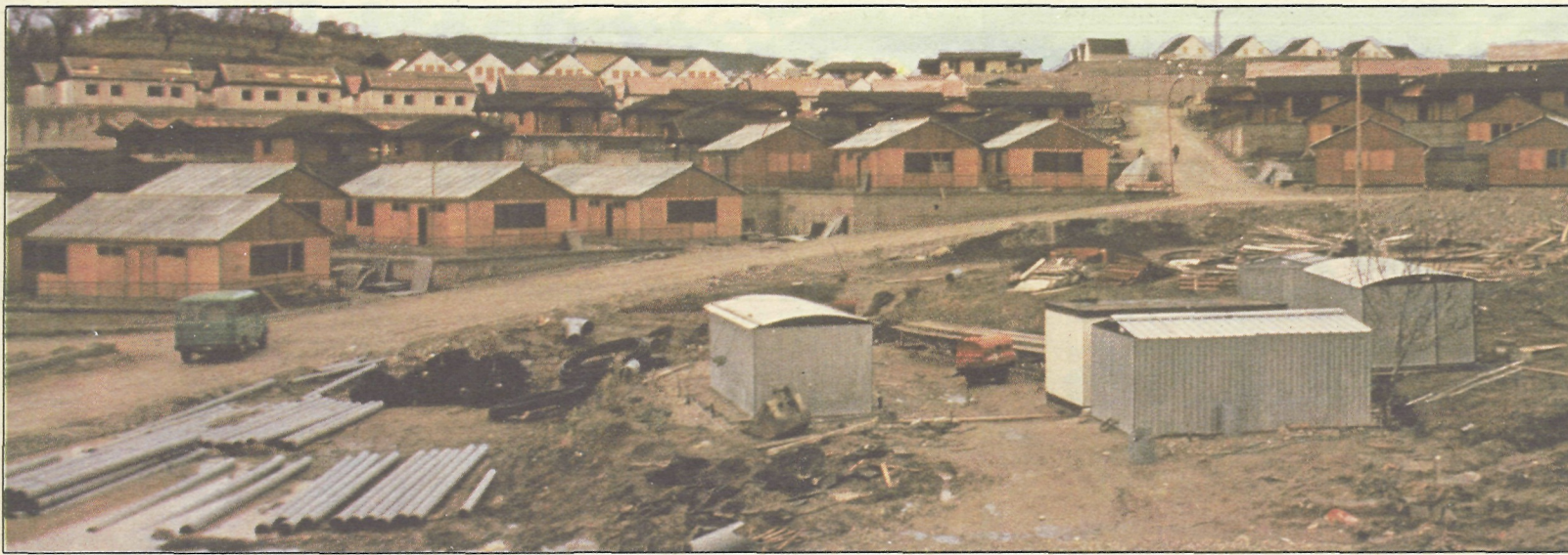
Known as "The Philadelphia Project," this reconstruction was generously financed by the Sons of Italy and the Archdiocese of Philadelphia
