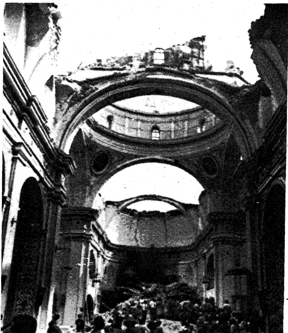
Church in Popayan, Columbia, hit by earthquake in March.
