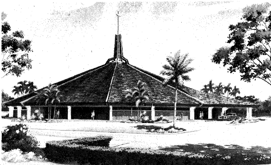
NEW CHURCH NEEDED —Holy Spirit Parish in Lantana has raised more than $1 million of $1.8 million needed to build a permanent church. According to Father William O'Dea, pastor, the area's rapid growth and projections for increasing population in the future make building the new church essential.
