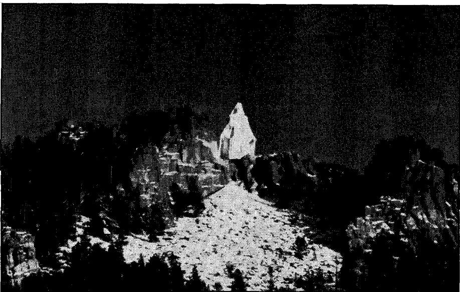
MOUNTAIN LADY - Finally assembled, the 90-foot steel statue stands on the Continental Divide overlooking Interstate 15 near Butte, Mont.
