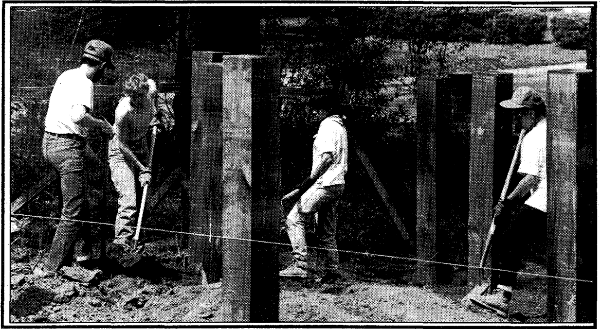
Students from UM build foundation of home for poor in Tallahassee.
